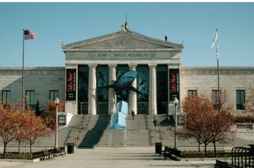
■ The John G. Shedd Aquarium was built for the Chicago Exposition in 1892, and before its renovation in 2004, the roof was a patchwork of different systems installed over the years. (Photo courtesy of EternaBond.)
